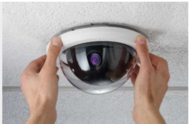
And replace the bubble.
