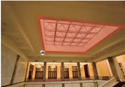
Skylight protection at Public facility / Warehouse
