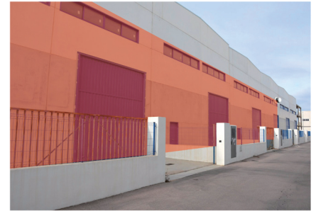
Wall protection (outdoor) at Warehouse
