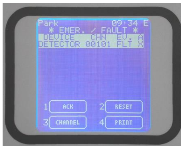
Fig. 3.2.1.d) Typical FAULT state of the ACTIVE EVENTS screen.
